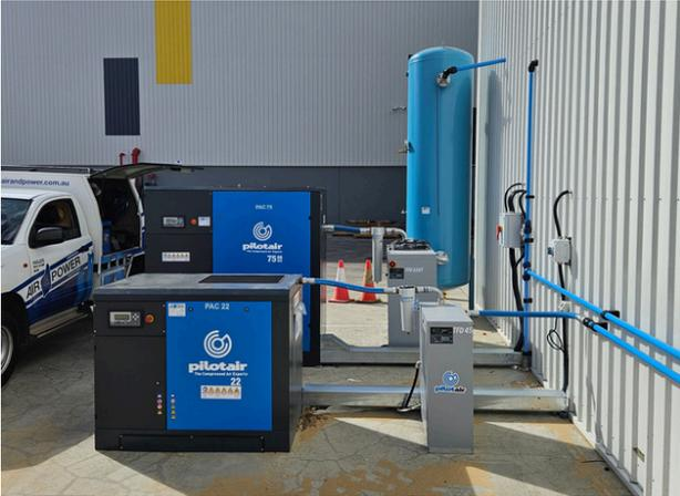
Pilot PAC75 with a TFD 220T air dryer and a PAC22 with a TFD45 Air dryer both with a 2150L vessel each, for **Expressway Spares' new workshop in Forrestfield.**
